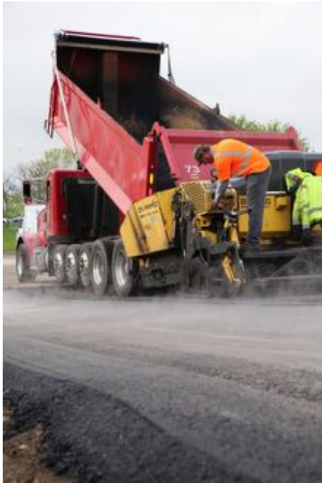
Road resurfacing in Hamburg
